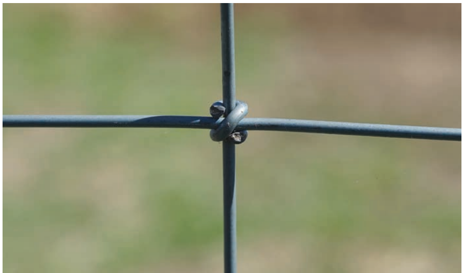
Square knot: The square knot is also commonly used in prefabricated exclusion fencing, and is found in Whites Wires Stiffstay, Southern Wire Farm Fence, Clipex S-fence and Waratah Stocksafe-T.
