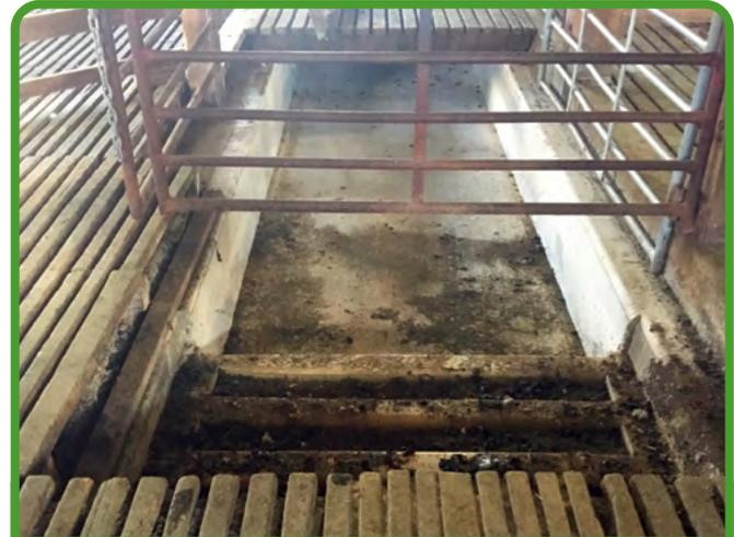
**Hidden solution:** Permanent concrete footbath under slats in shearing shed. When the footbath is not in use, the grating sits back over the footbath allowing for normal use of the shed.
