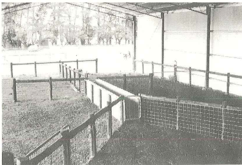
Photo 13. Steel mesh used in conjunction with treated timber posts and rails.
