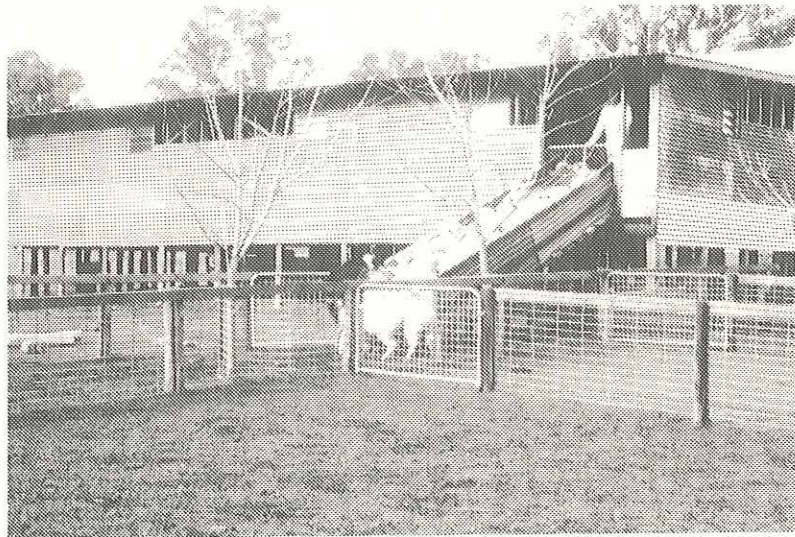
Photo 12. Yard fences using timber and steel components.
