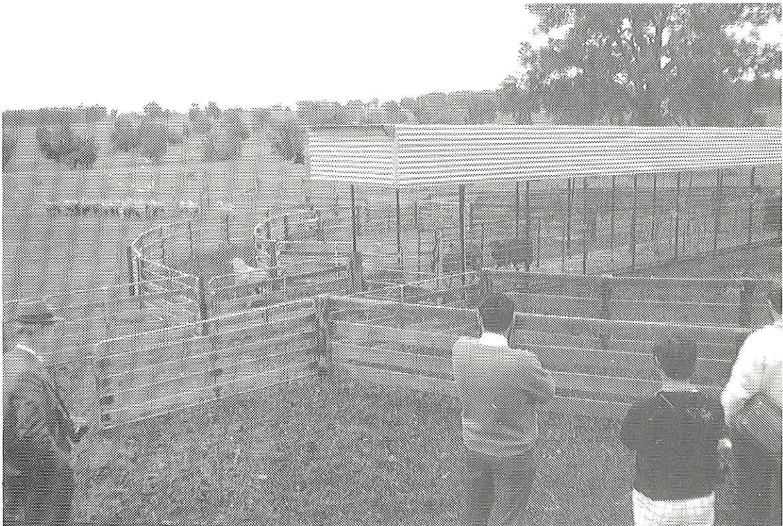
Photo 3. End of the working race showing the circular laneway connecting the holding areas with the working area. Note also the large gates available to direct the flow of sheep.
