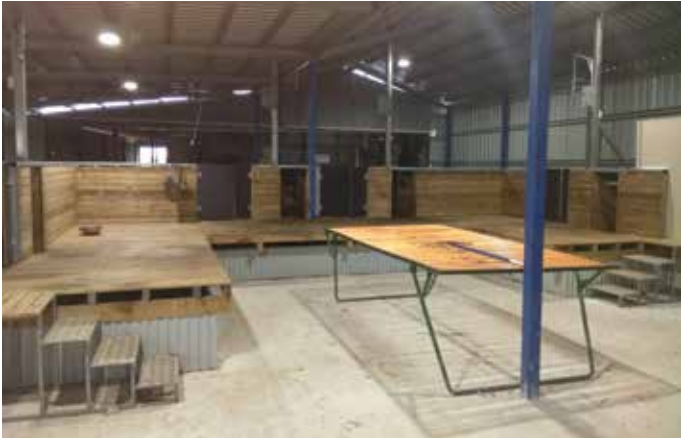
Figure 7: wool room and board with minimal distance travelled by shed staff. Don since has added handrails at the stairs to the raised board, running 900mm above each step.
