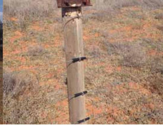
Figure 3: A close-up of the poly insulators installed.
