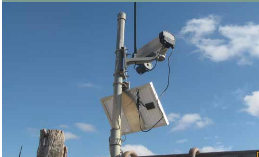
Figure 3: Smart Water telemetry system.
