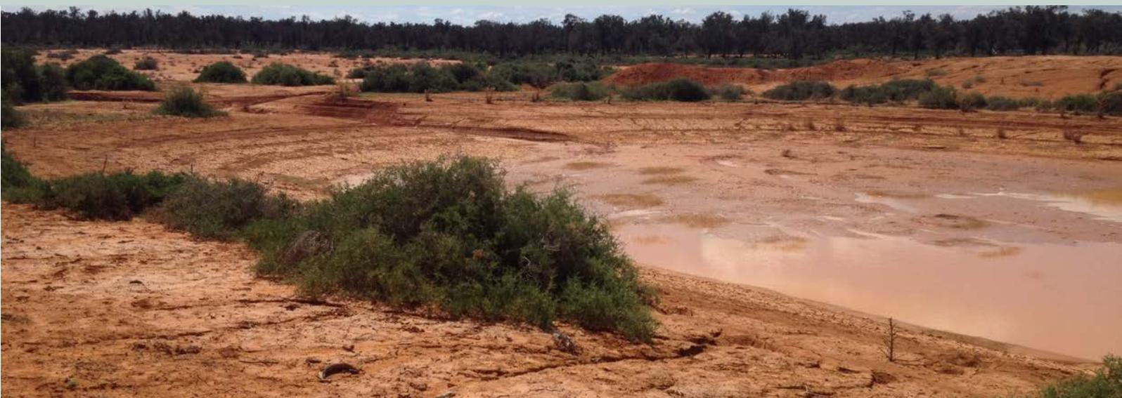
Figure 4: Water entering the silt trap and settling before it is pumped to the Superdam.
