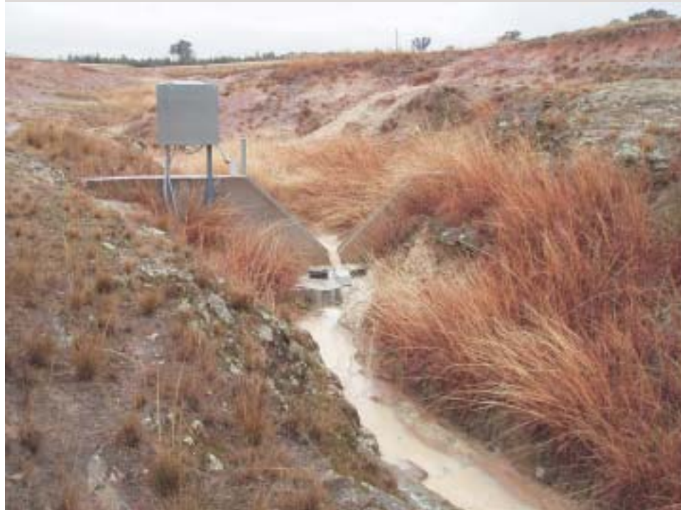
Monitoring stations like this one have been constructed at the entrance and exit of a large gully on 'Bogolará', so that the effects of management on flow, sediment, and nutrient movement from the gully can be measured over time.
