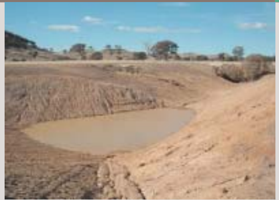
A large dam has been built near the head of the gully to prevent further erosion of the bed lower down, and to provide a valuable farm asset. Photo Fleur Flanery.
