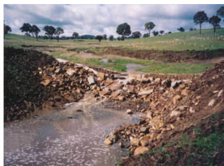
Above (before) and below (after)—Gully erosion, controlled with a cheap erosion control structure, battering of steep banks, a concrete weir, rocks to take the impact of falling water, fertiliser and pasture seed, tree and shrub planting, and stock exclusion. Photos by Caroline Street.
